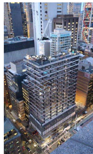
20 Martin Place stripped back to its steel frame. Photo: Built
